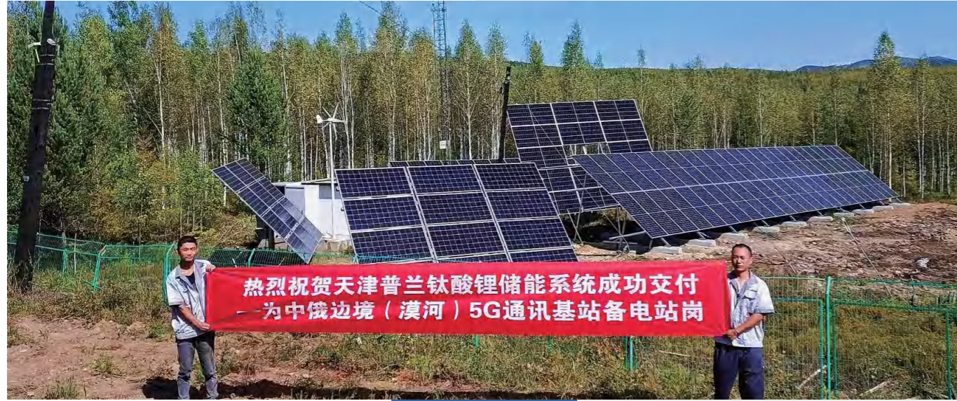
Heilongjiang | 5G communication base station backup power | 2MWh
