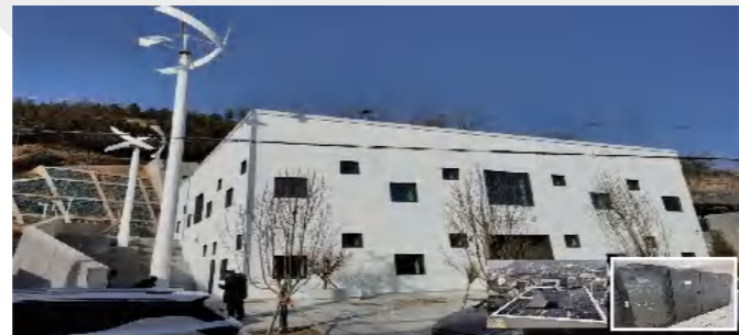
Gansu | Wind and solar energy storage and charging microgrid | 400KWh
