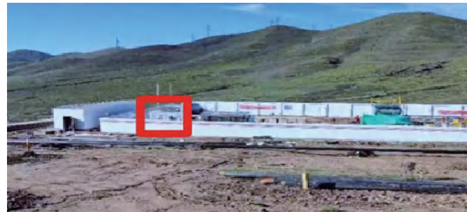
Qinghai | Natural gas plant station energy storage project | 386.4V/192Ah
